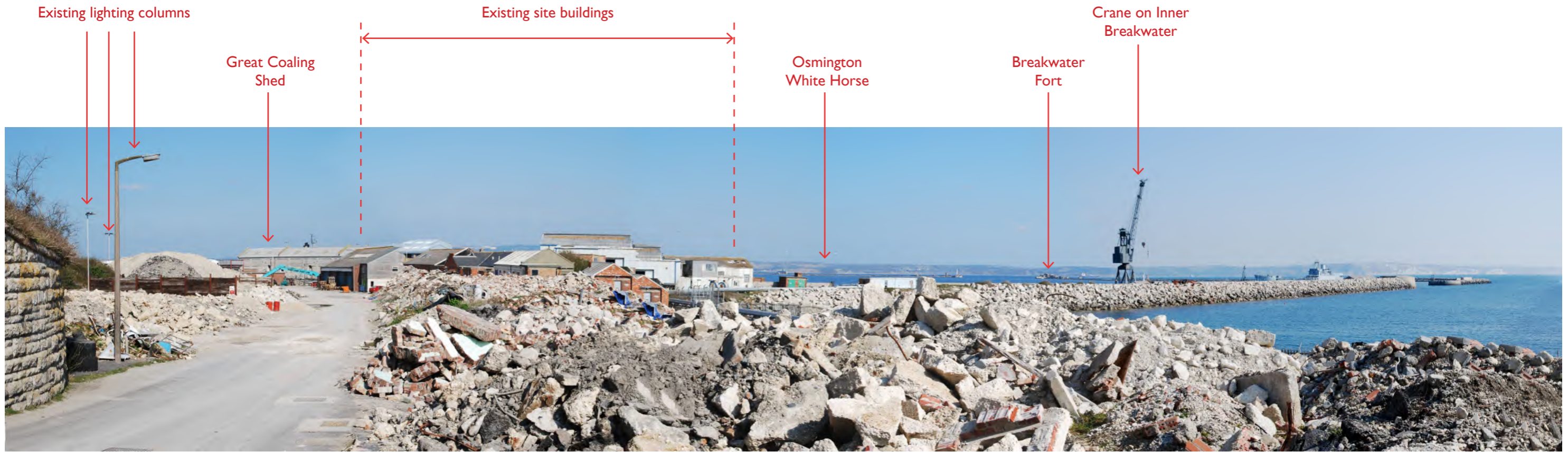
Viewpoint A: From From southern edge - looking north west
