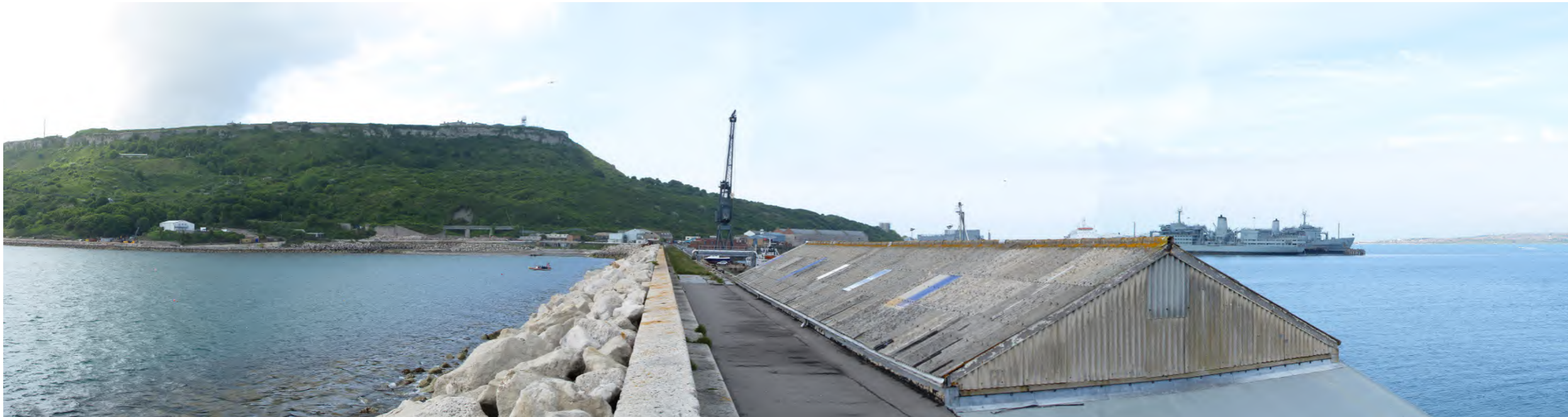
From the end of Inner Breakwater, looking south west - View 3 (Existing)
