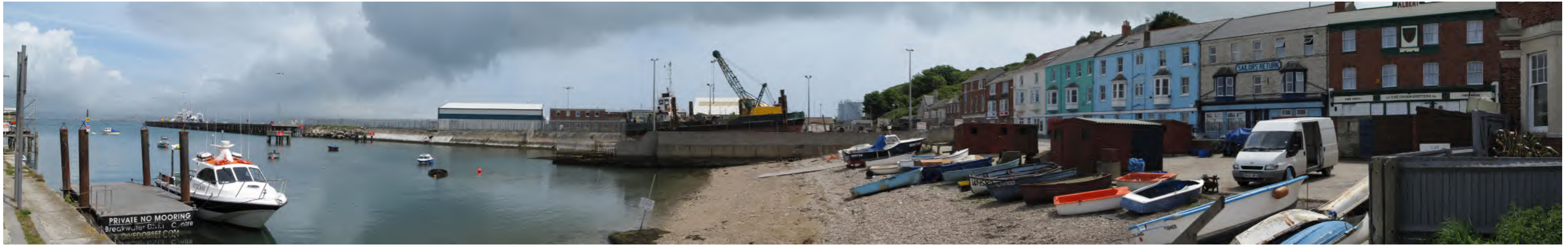
From Castletown Pier, looking east - View 4 (Existing)
